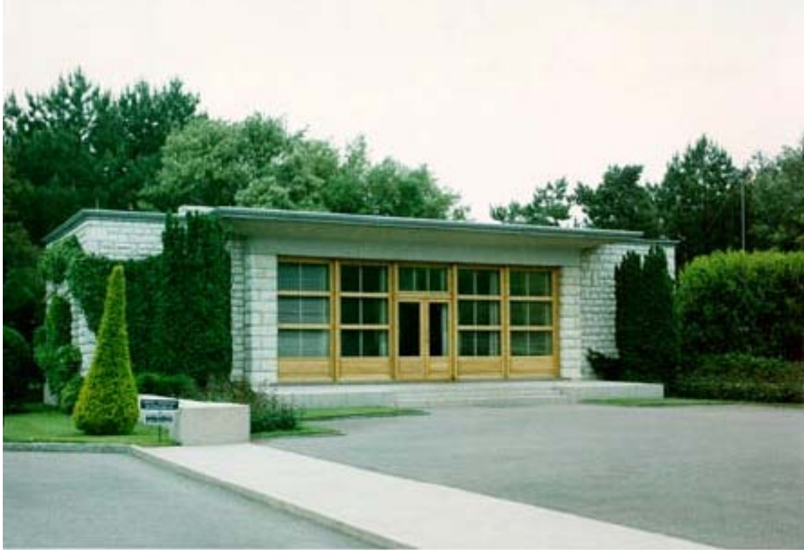
Exterior of the Visitors' Building
